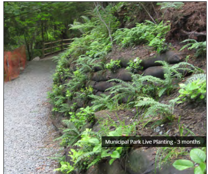
Figure 15. Mechanically Stabilized Earth, Three Months After Planting. Credit www.flexmse.com
