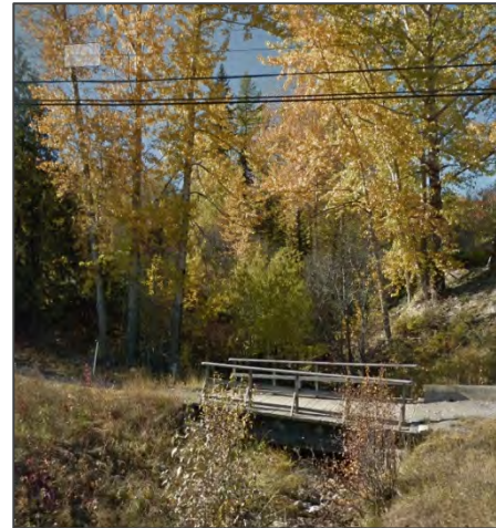
Figure 17. Existing Brydon Creek Bridge that will need to be Upgraded.
