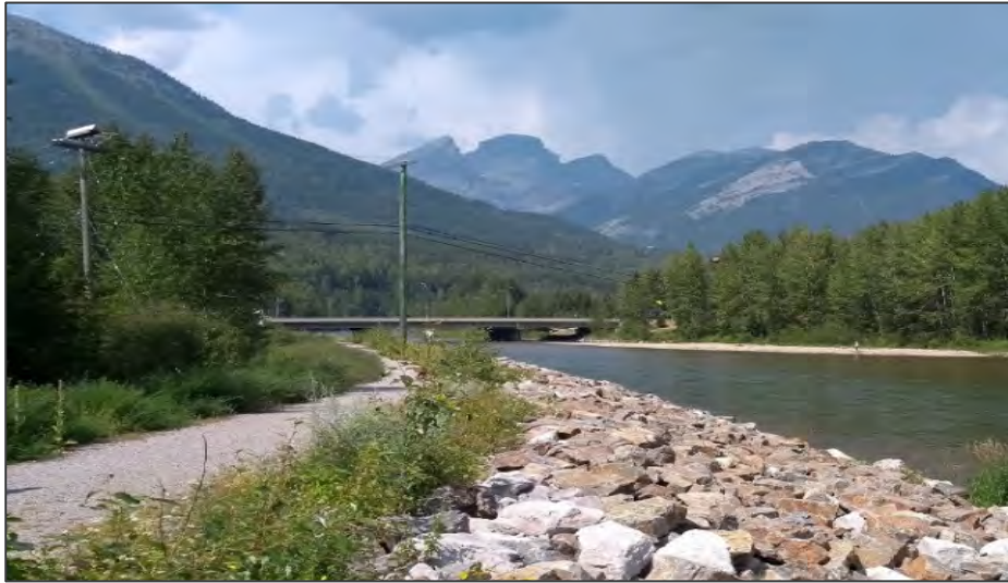
Figure 4. Existing West Fernie Dike Trail Downstream of the West Fernie Bridge.
